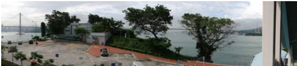
A Panoramic View of both Ting Kau Bridge and Ching Ma Bridge
